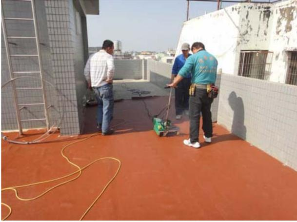
A photograph showing a worker on a rooftop terrace using a self-propelled welding machine to weld the waterproofing membrane. The worker is wearing a blue shirt and dark pants. Another worker is standing nearby. The membrane is reddish-brown and covers most of the terrace.             |
