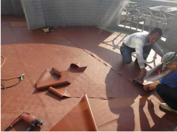
A photograph showing two workers on a rooftop terrace. They are in the process of laying a reddish-brown waterproofing membrane. One worker is kneeling and using a tool to secure the membrane, while another is standing nearby. Several sheets of the membrane are scattered on the ground.  |
